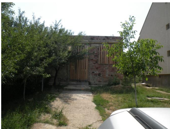
Figure 15. Former heating point–before
