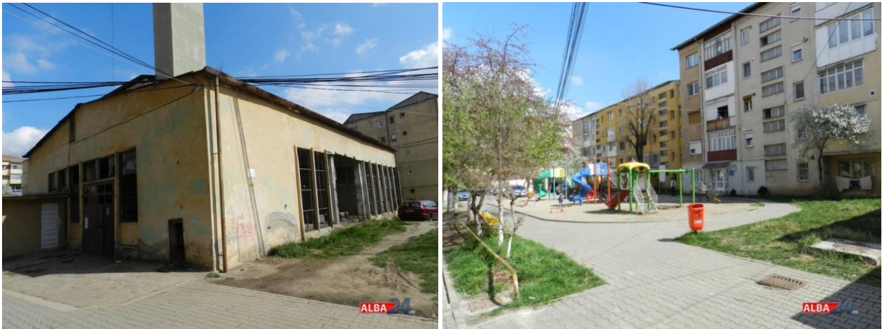
Figure 2. and Figure 3. An abandoned heating point in Alba Iulia city located near a playground
