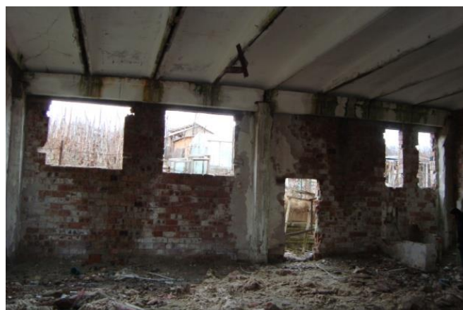
Figure 16. Former heating point–before
